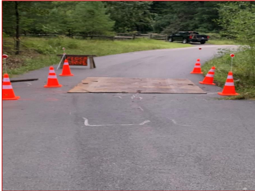
View from Audubon Rd. of temporary steel plate on Maverick Rd.
