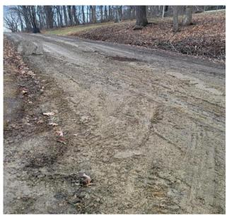
This is what happens when salt is applied to unpaved dirt/gravel roads. NEVER APPLY SALT TO UNPAVED ROAD SURFACES!
